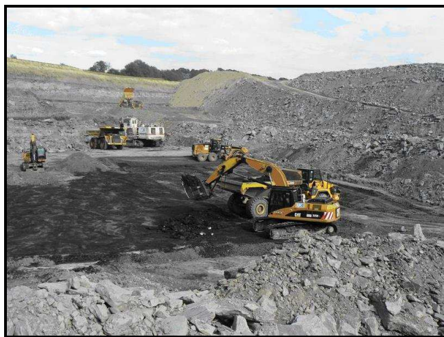
Figure 1: The large 'digger' at the back removes the bulk of the spoil, the small digger in front scrapes off the last layer exposing the coal bed for mining
