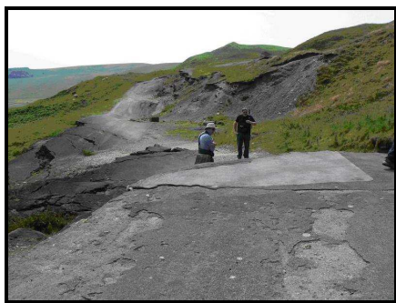
Figure 3: Landslip at Mam Tor.
