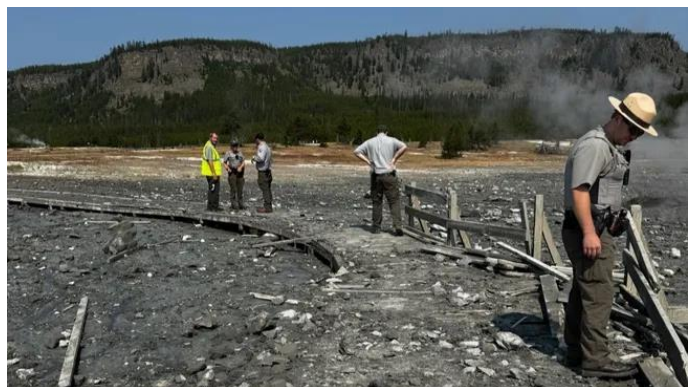
Yellowstone National Park staff assess the damage to Biscuit Basin boardwalks after a hydrothermal explosion on Tuesday (July 23). (Image credit: National Park Service)
