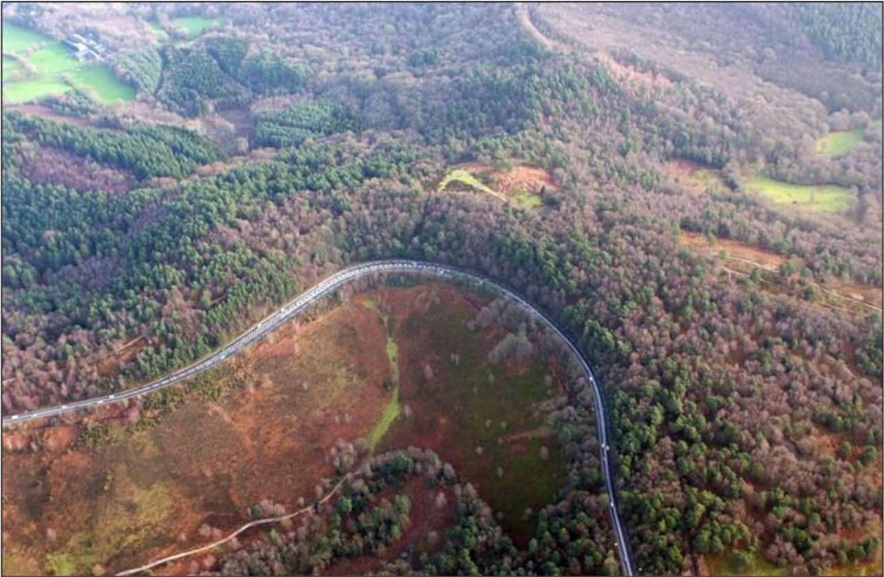
Aerial view of Devil's Punch Bowl (photographed in January 2007, before the closure of the old A3). (Credit: Highways Agency)
