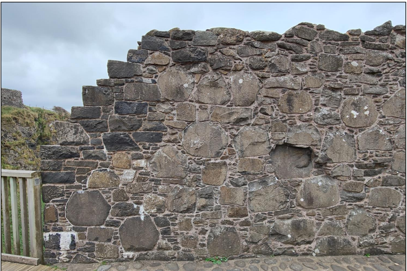
Figure 1-5. Building blocks within the castle walls made from columnar basalt.
