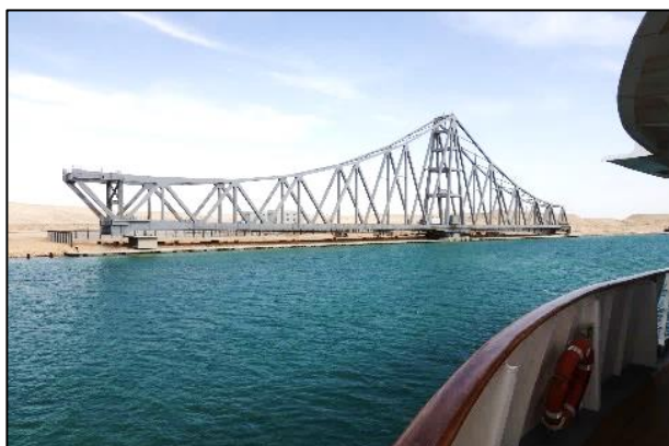
Figure 4: Railway swing bridge.
